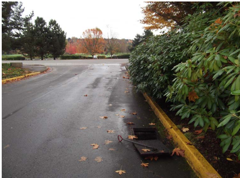
Flows are directed through the parking lot via the business park's storm system. Flows enter this catch basin just beyond the quarter mile buffer. Willows Rd NE is visible in the background of the photo.
